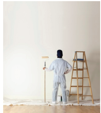
The wall is being painted.
